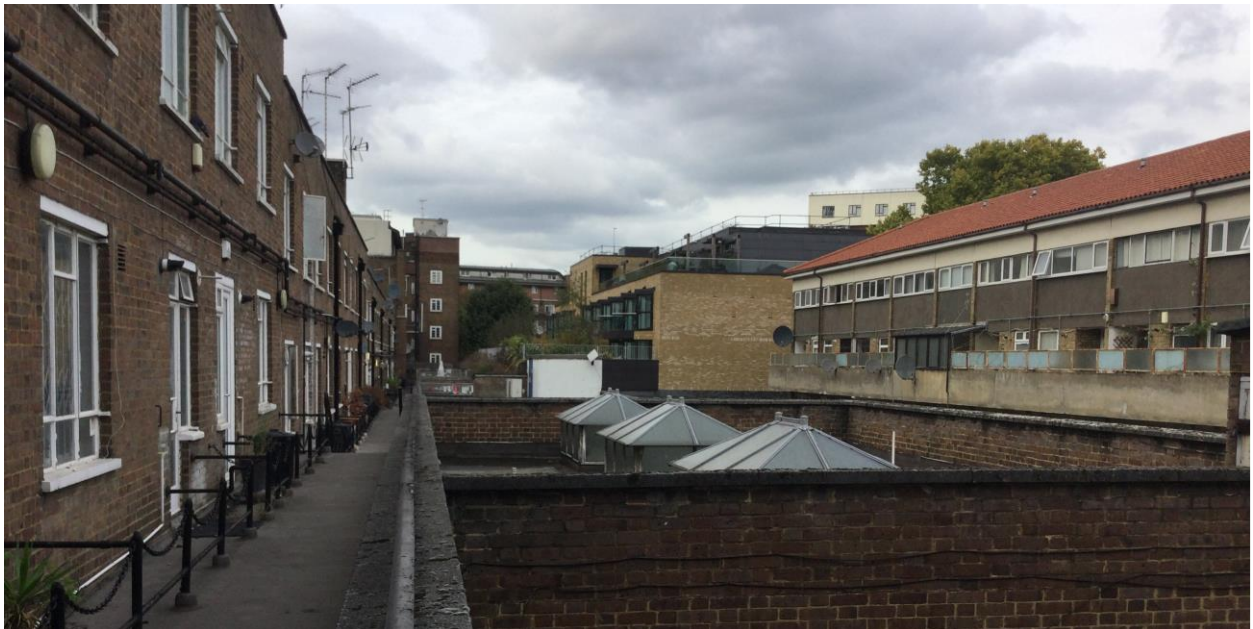
Rear of the application site – looking towards Cervantes Court and Aird House
